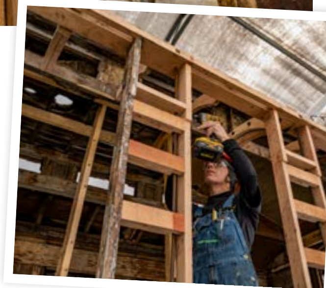
Jenni Mack, Carpenter, installing framing. > Photo by Jerry Day
